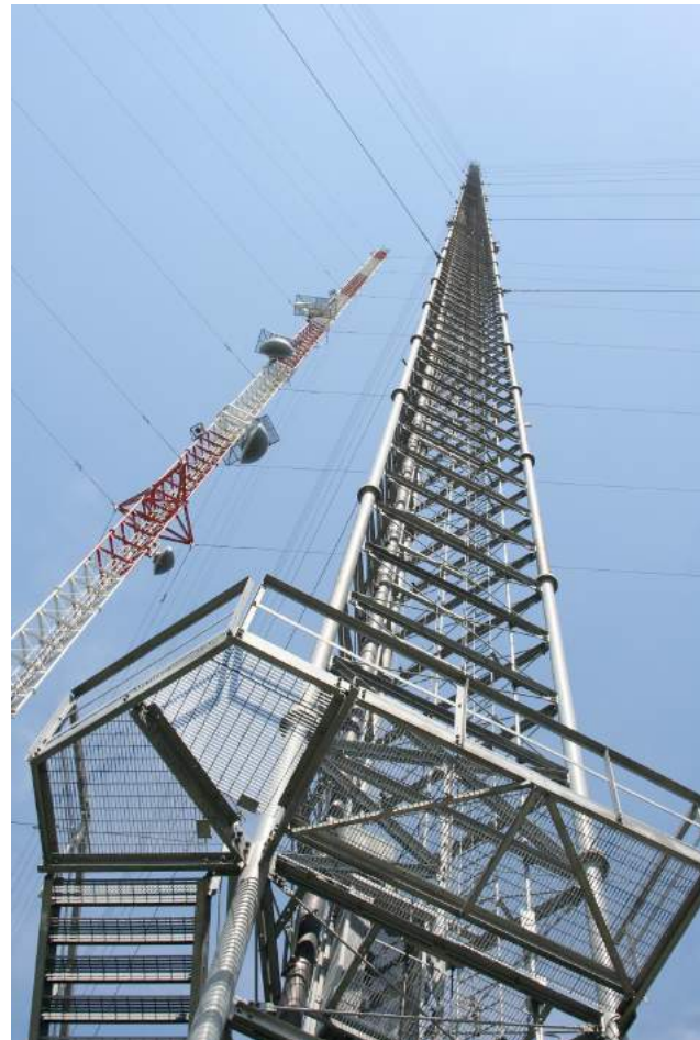
FIG 1. The transmitter tower for WXP-TV.
