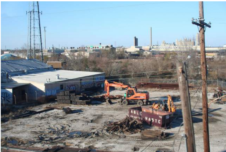
FIG. 3: Duckworth-Dunn's scrap metal processing facility
