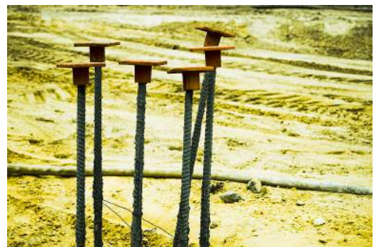
FIG. 2: An example of capped rebar at a construction site.
