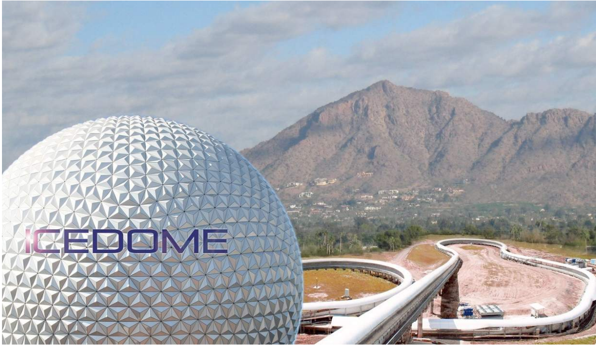
FIG. 3: Exterior of IceDome, near completion. The Iceway bobsled/luge track is at right, with the primary dome structure at left.
